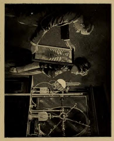
Modern Improved X-Ray Apparatus Showing Mica Disk.
